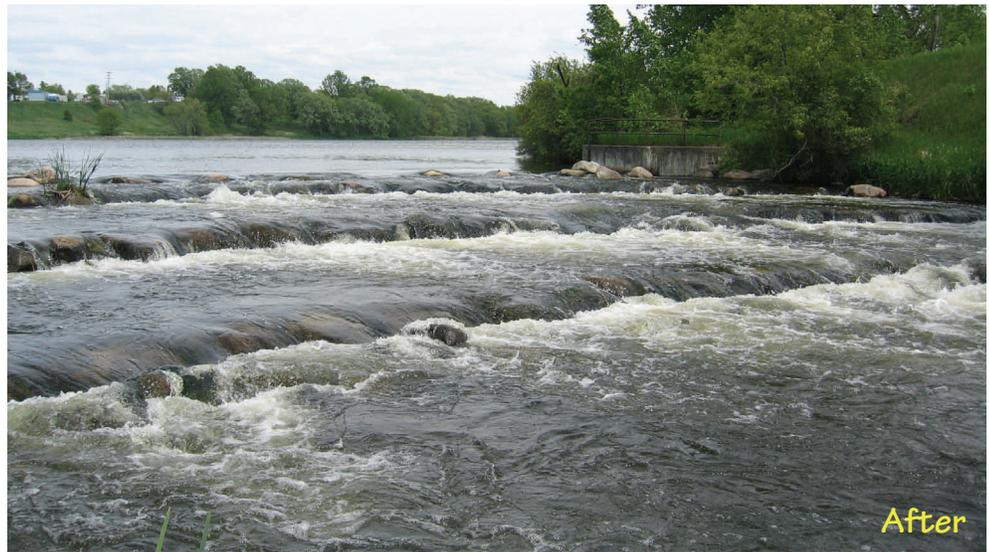
*Dams throughout Minnesota are being removed or modified into a stone rapids as a means of restoring stream health. This approach restores the natural flow of the river, allows the fish community to migrate upstream, provides spawning habitat, removes the drowning hazard, and provides recreational opportunities.*
