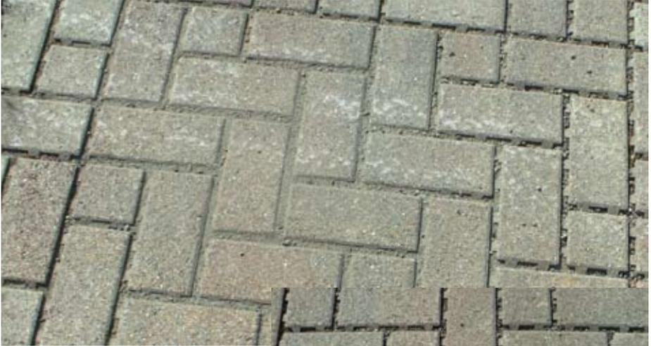
Above is a picture of pervious pavers that have not been properly maintained and the sediment has filled up to the tops of the pavement.
