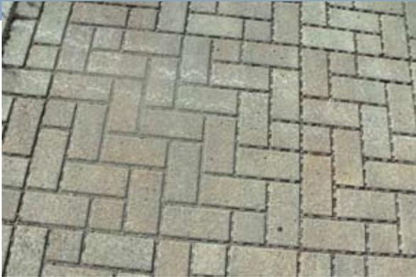
The picture to the left demonstrates what sediment accumulation can look like. These pervious pavers no longer function.
