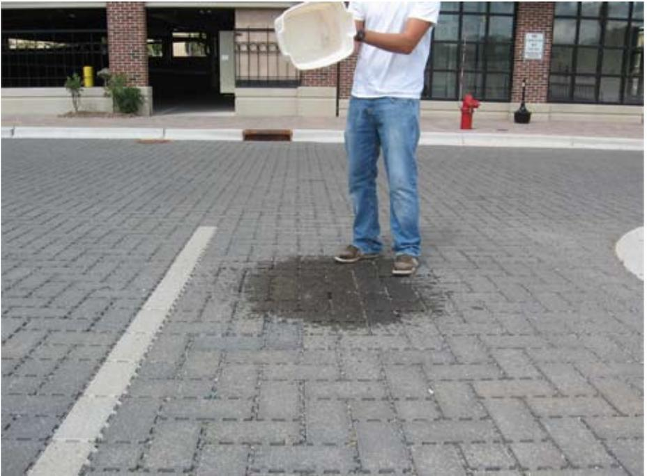
These pavers are still working properly. The water drains directly down into the storage chamber below instead of running off.
