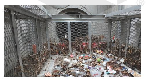
Nutrient Separating Baffle Box with collected trash, organics and debris inside the screened basket system ready for disposal.
