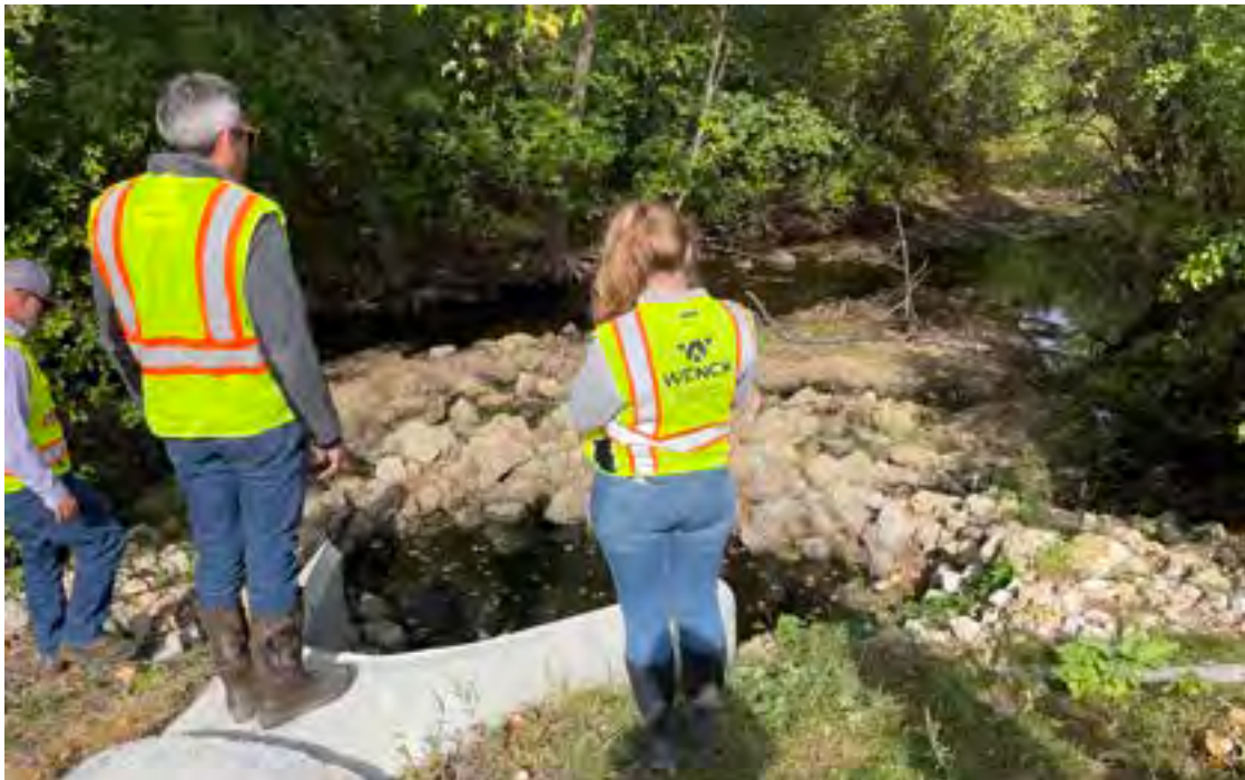
Figure 5: Outfall along connection corridor.
