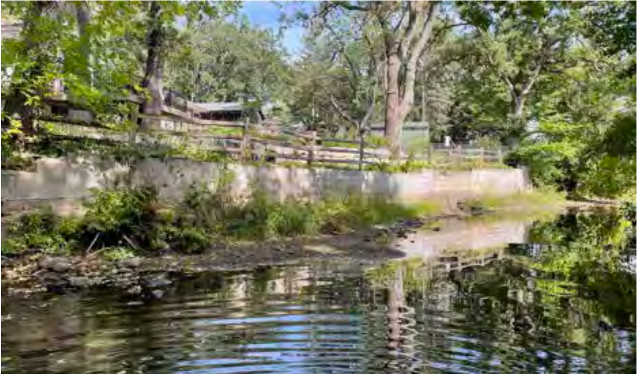
Figure 3: Cinderblock wall downstream of utility crossing.
