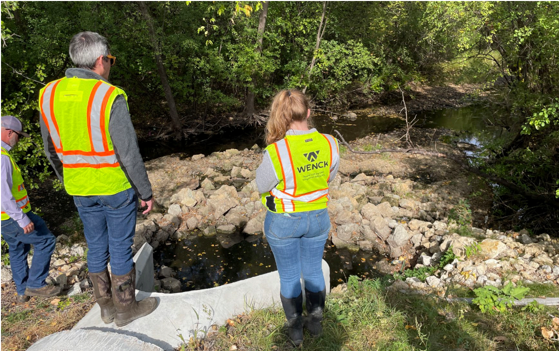
Figure 5: Outfall along connection corridor.
