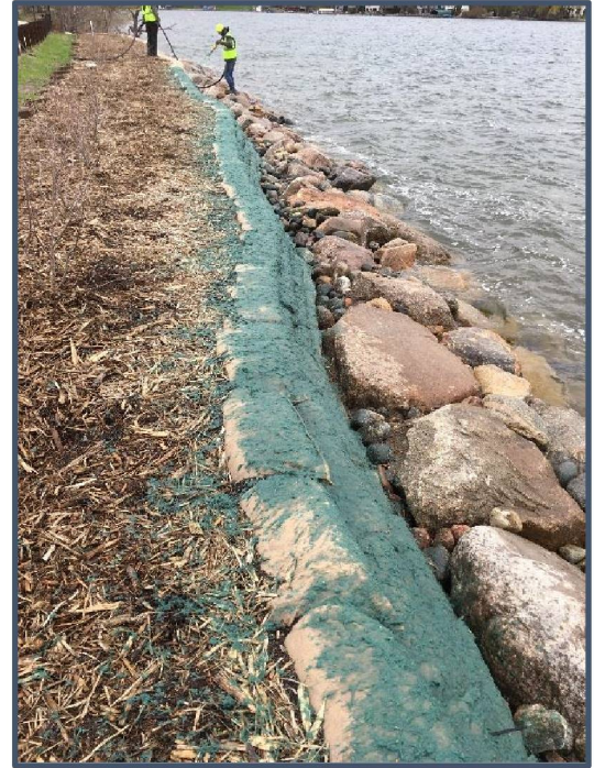
Hydroseeding the Bushaway Road soil slope, April 27
