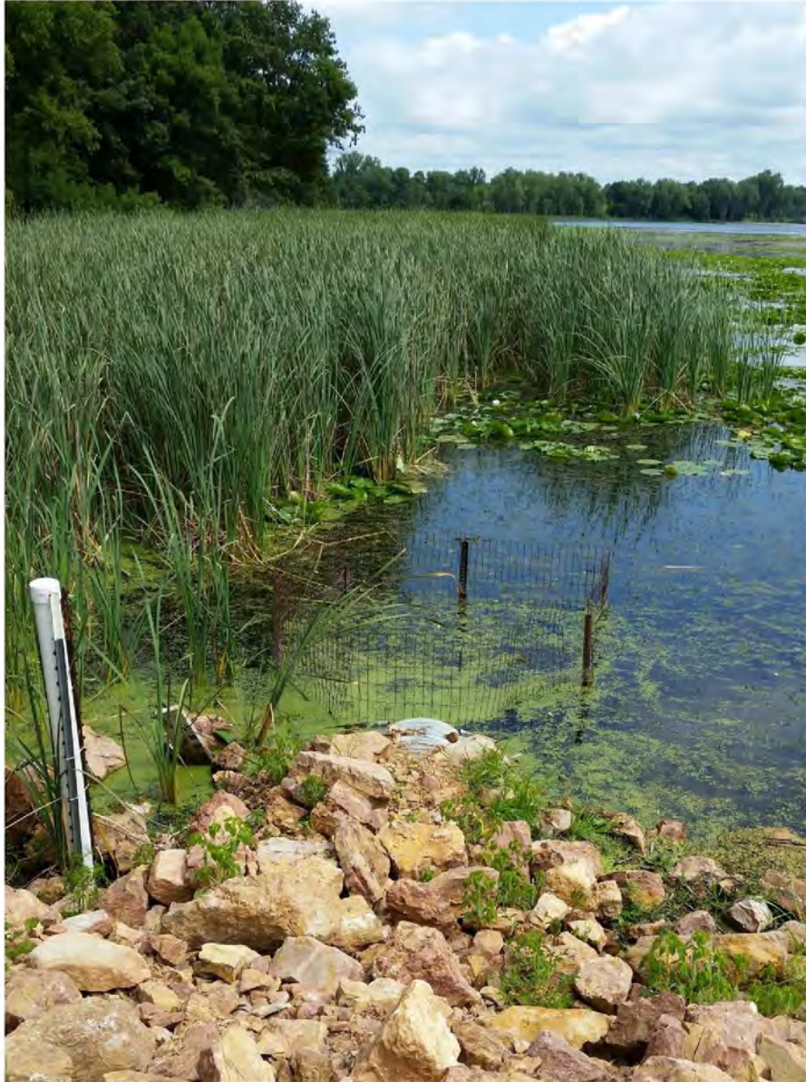
Figure 36. A photograph of the barrier in place at the Zumbra Lake outlet to Sunny Lake in the Carver Park Reserve. Lake levels were observed overtopping this barrier in August of 2016.
