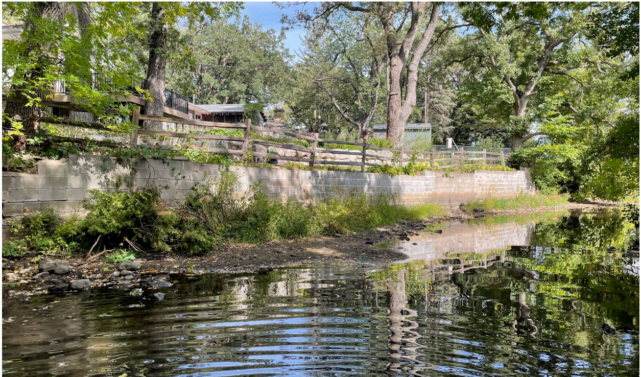
Figure 3: Cinderblock wall downstream of utility crossing.
