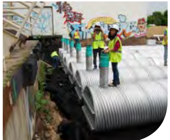
Underground stormwater treatment in Minneapolis
