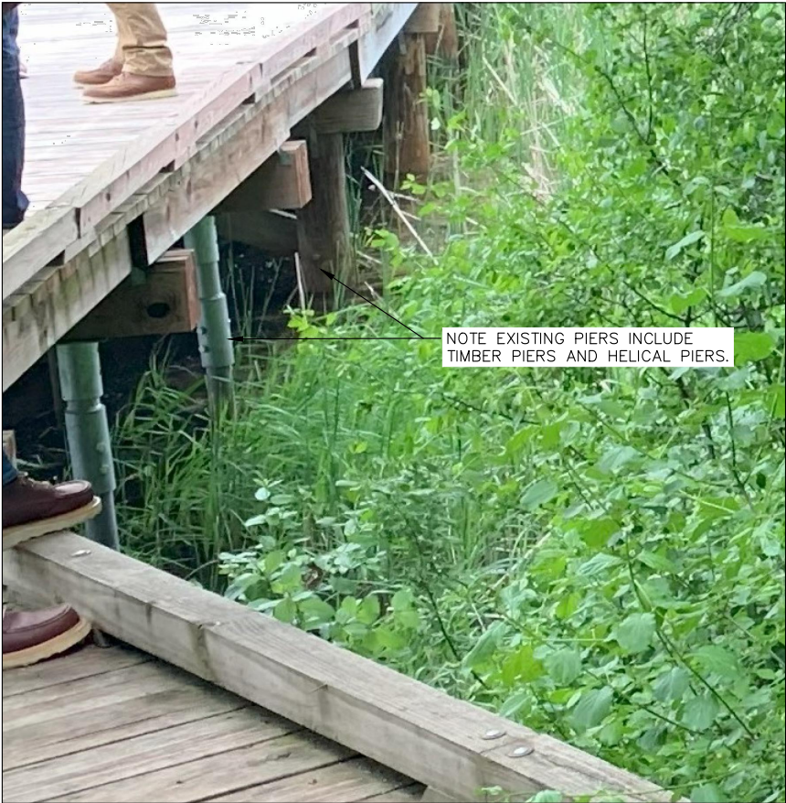
PHOTO 3: TIMBER AND HELICAL PIERS
