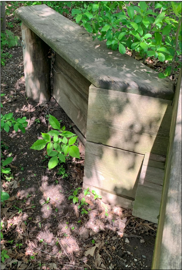
PHOTO 2: EXISTING ABUTMENT
