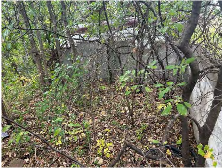
Photo #5 View of former building footings/wall on south side of farmstead toward Painters Creek.
