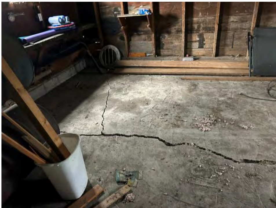
Photo #16 View of concrete floor in one of the wood sided sheds.
