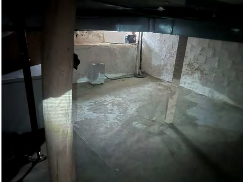
Photo #11 View of residence basement with sump pit in background.
