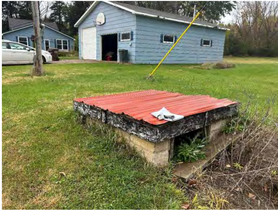
Photo #7 View of unused water well pit/cover in foreground with garage and residence in background.
