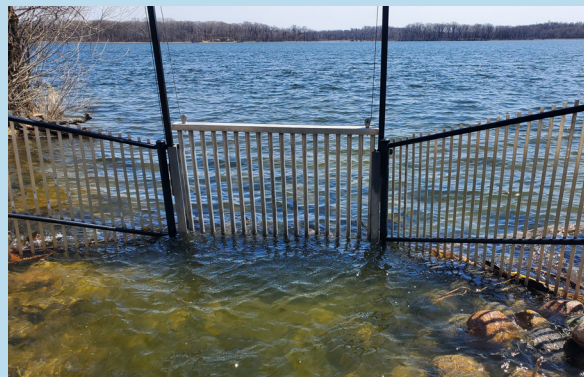
A barrier at the outlet of West Auburn Lake prevents carp migration from a productive nursery.
