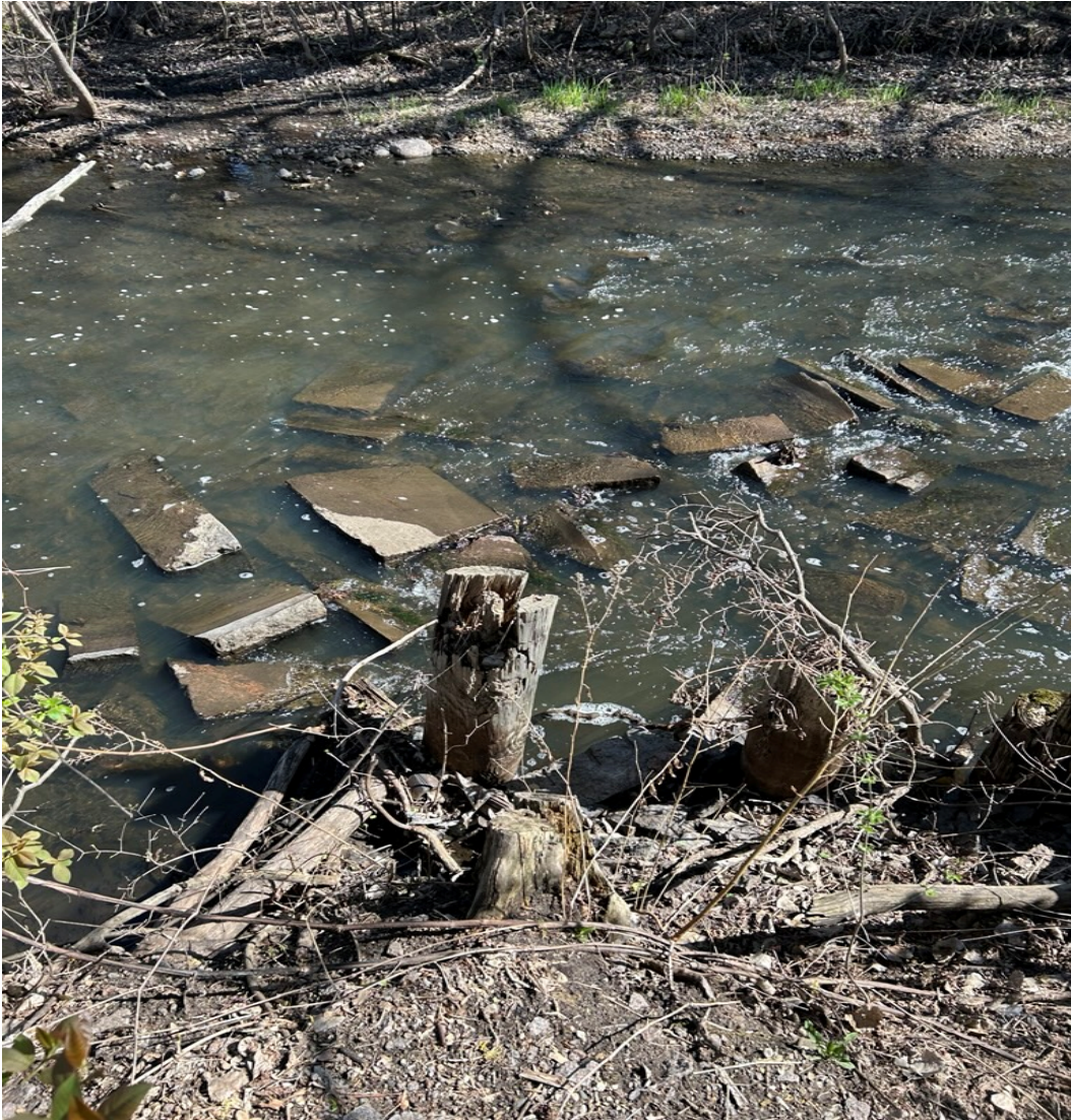
Image 4. Old Railroad Spur Abutment (Geocell Bank Location)
