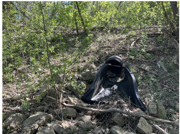
Photo 28. View of culvert outlet at upland point PP10. Photo taken facing east.
