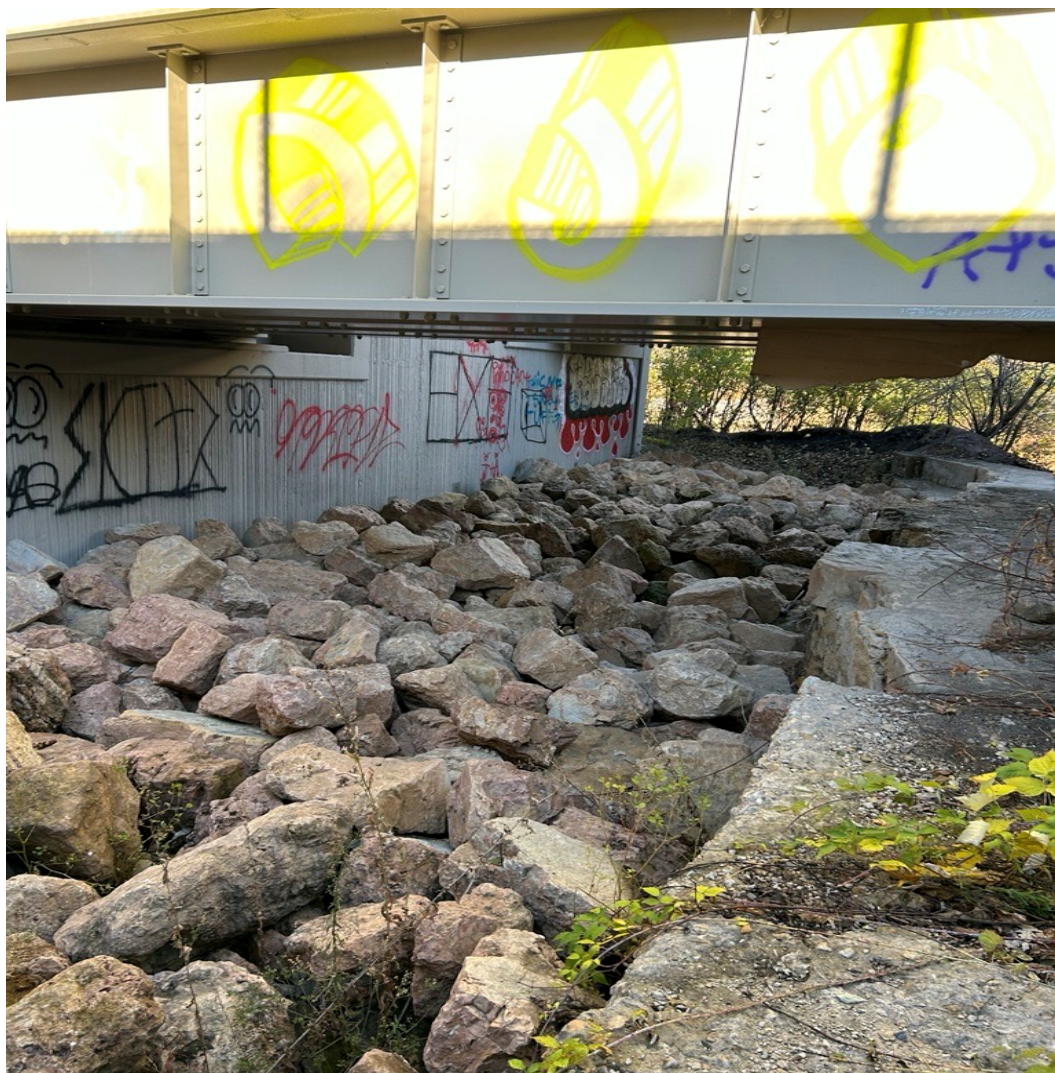
Image 1. Riprap Under Bridge
