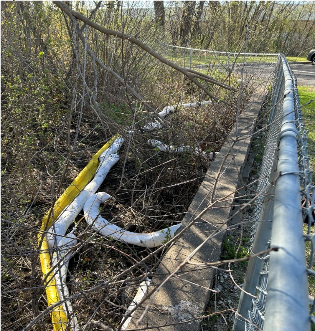
Image 9. 7800 Powell Road Retaining Wall
