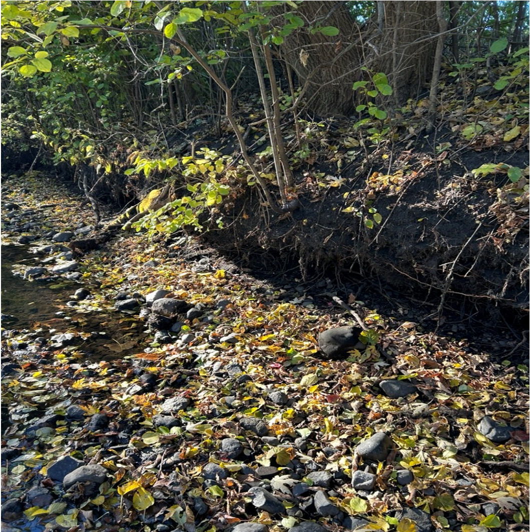
Image 5. Eroding Bank Downstream of Bridge (FES Lift Location)
