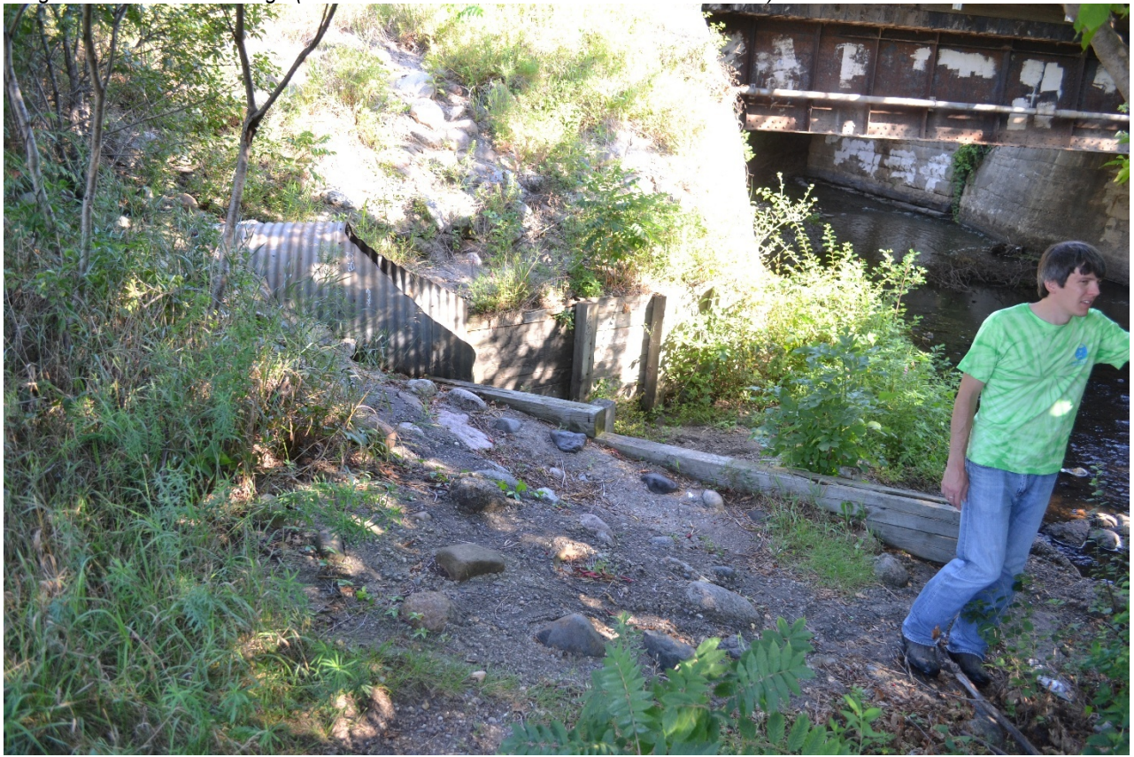
Image 6. Bank south of Bridge (48" CMP Outlet Location – MCWD 2012 Site Visit)
