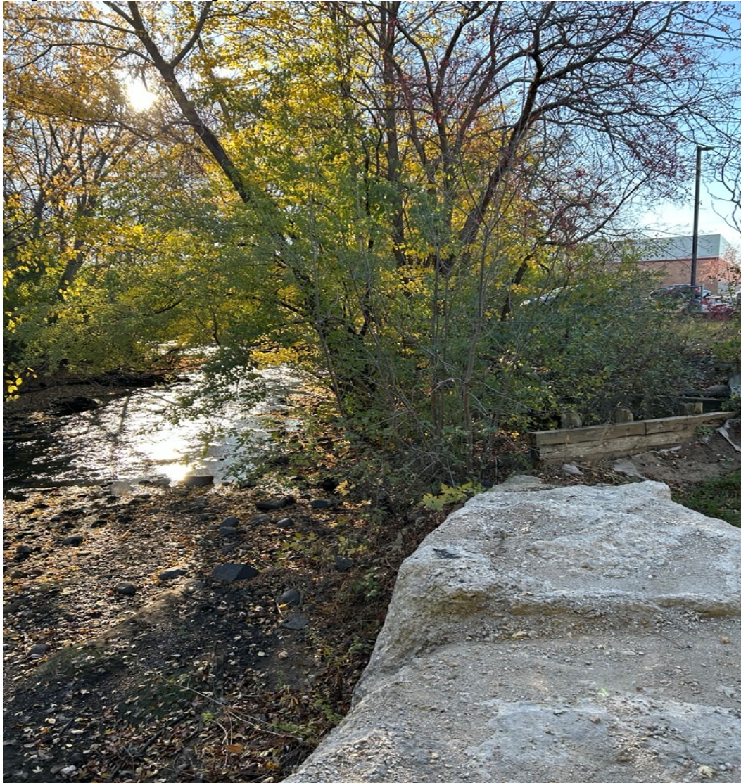
Image 7. Bank south of Bridge (FES Lift Location)
