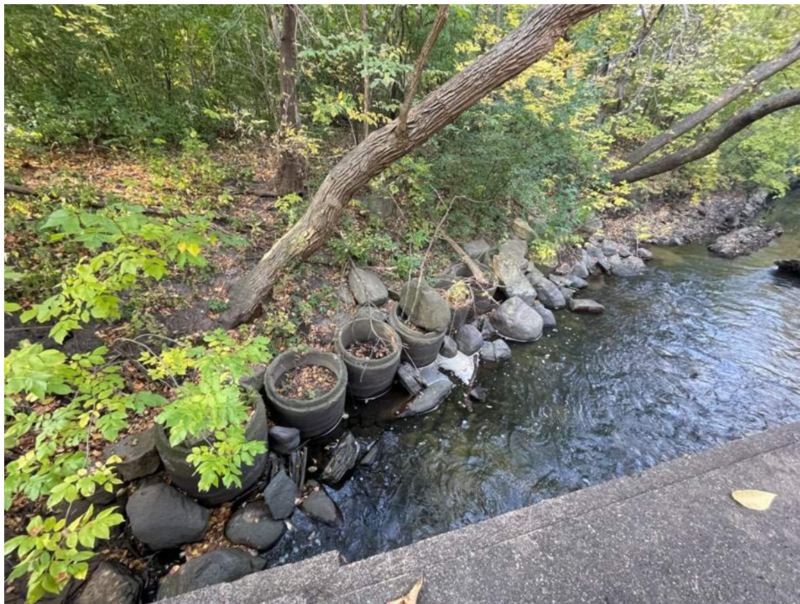
Figure 5. Vertical concrete pipes along stream bank upstream of the former parkway bridge. OCTOBER 10, 2024. Photo credit Maren Hansell
