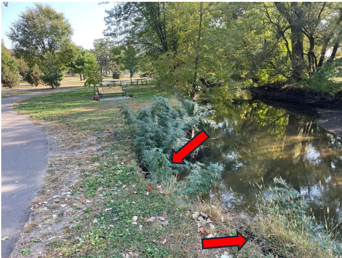
Figure 6. Outside bank erosion on the west end of the reach with new sitting bench installed. OCTOBER 10, 2024. Photo credit Maren Hansell
