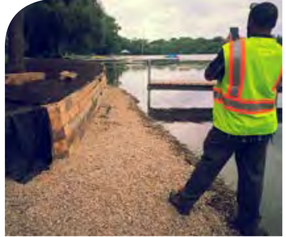
Staff inspecting a retaining wall
