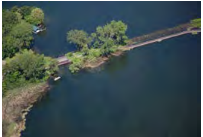
Gray's Bay Dam
