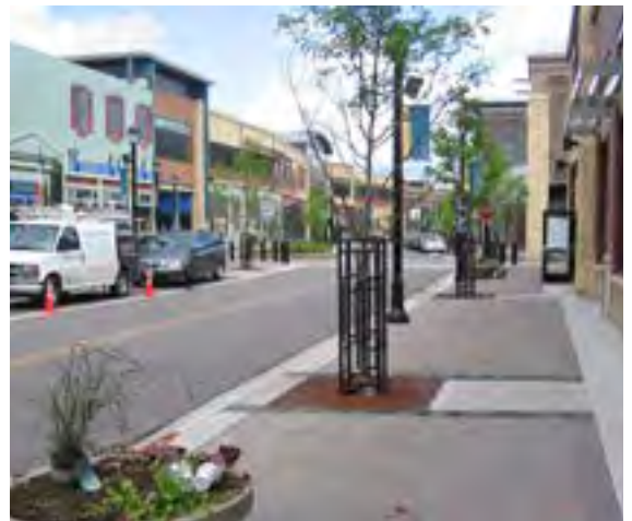
Low impact development practices in St. Louis Park
