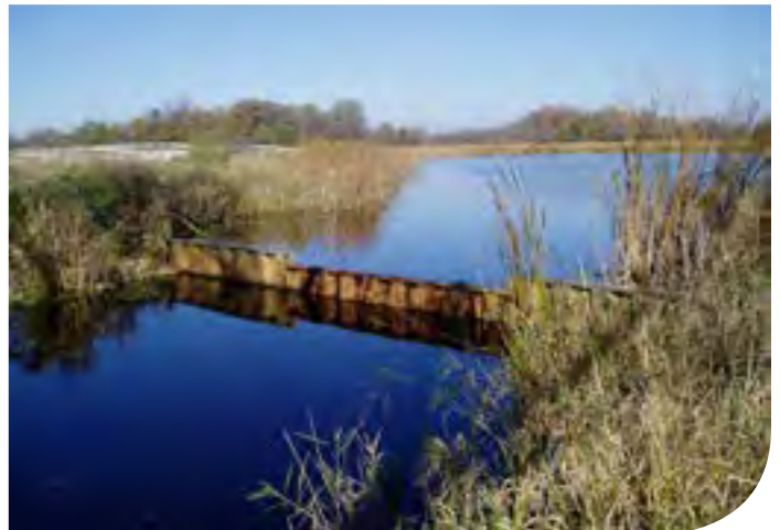
Painter Creek weir
