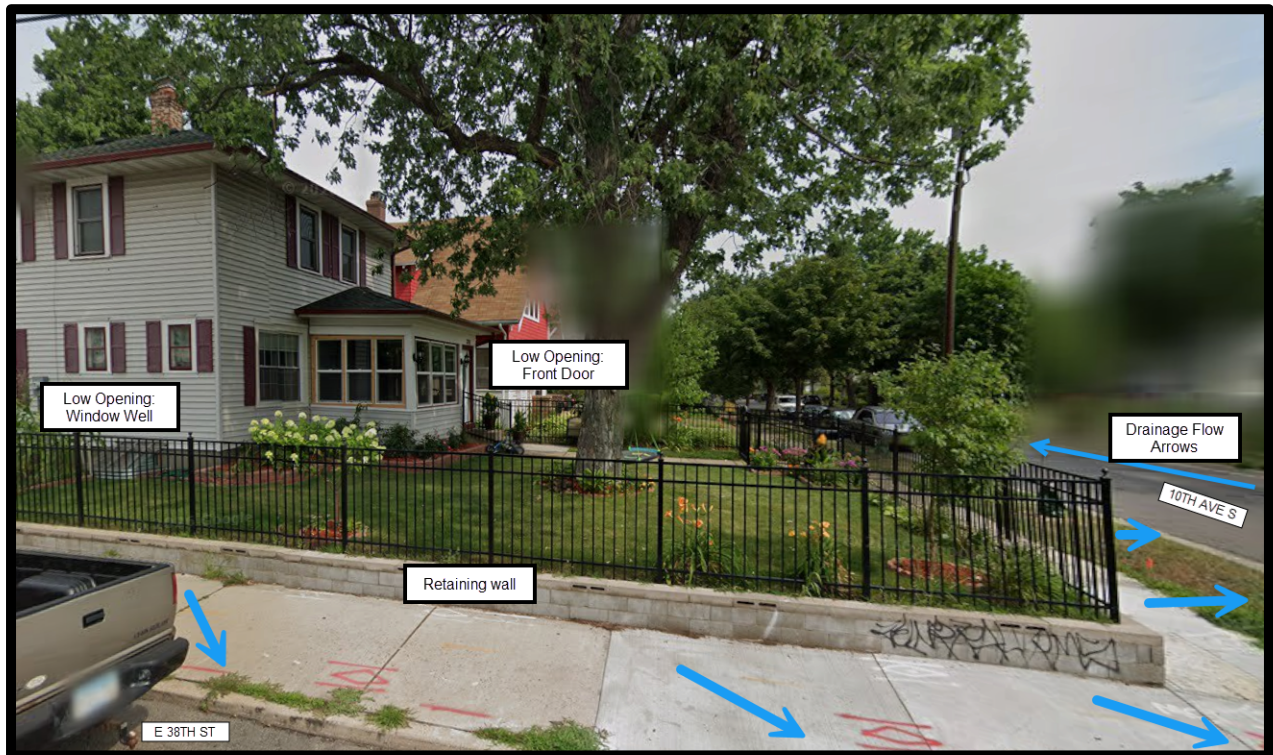
922 County Rd 38 Residence Low Opening & Runoff Pattern
