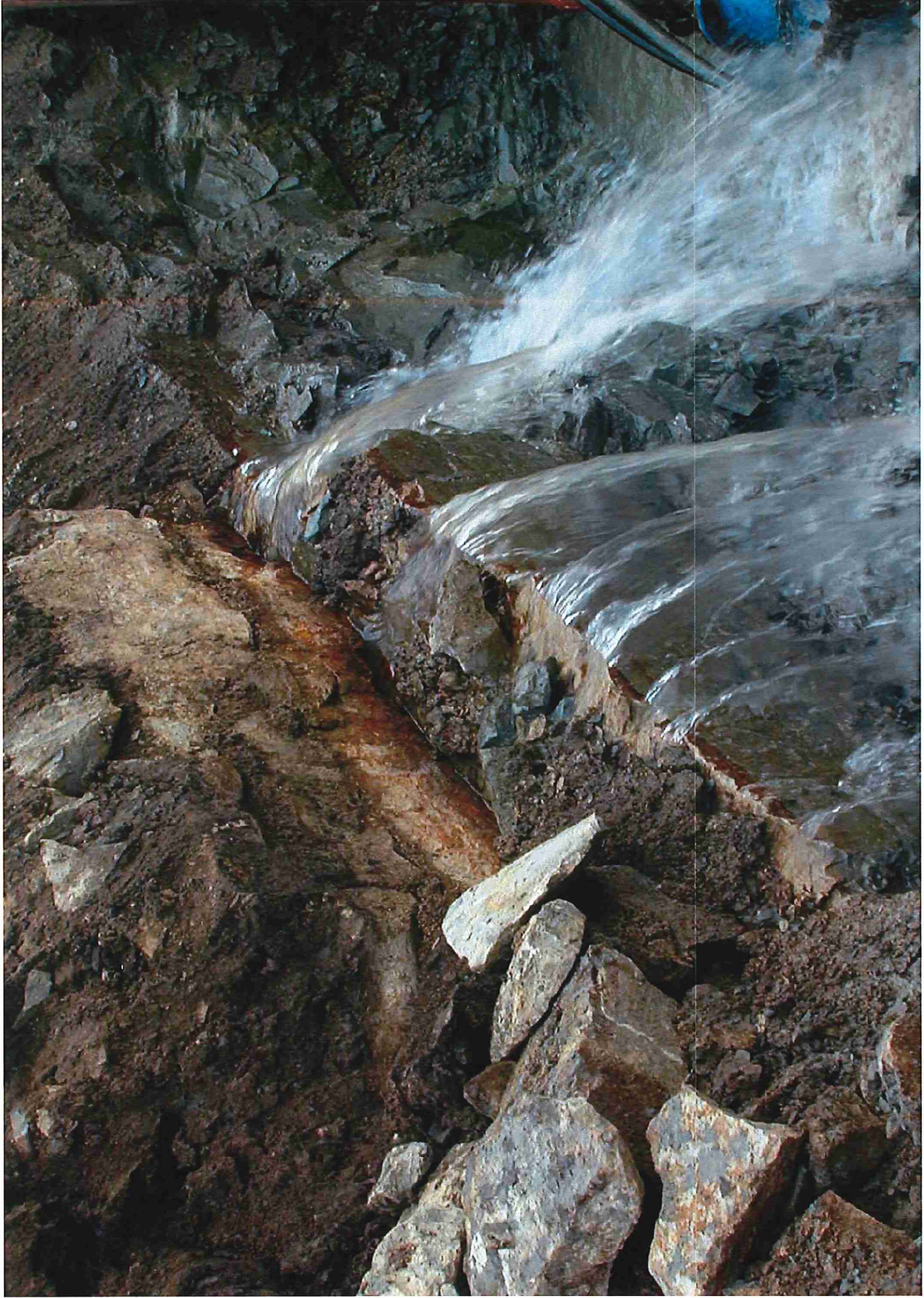
Figure 7. Groundwater entering excavation via basal Magnolia parting (photo by K. Barr)
