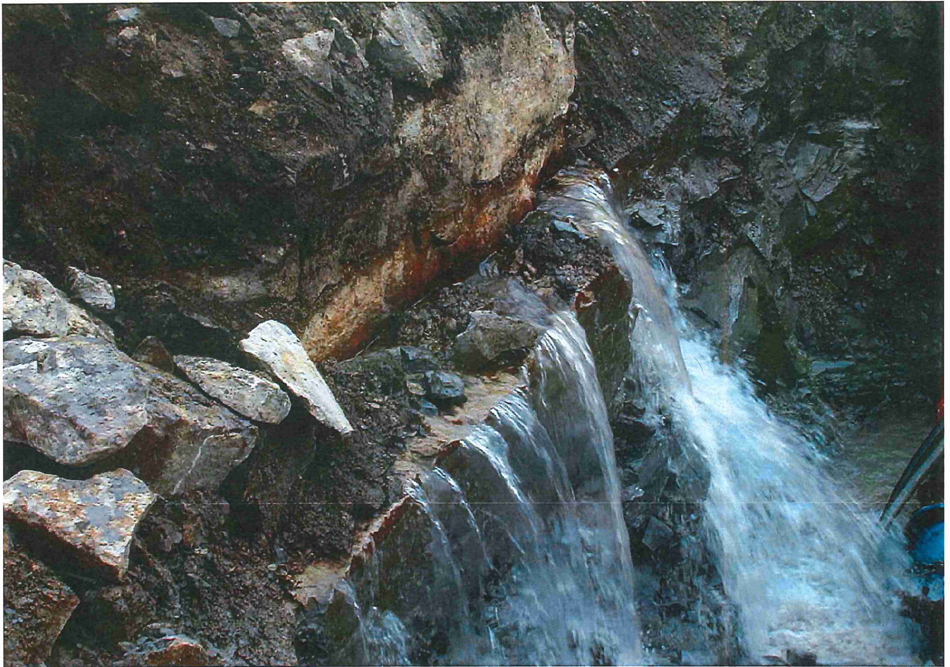
Figure 7. Groundwater entering excavation via basal Magnolia parting (photo by K. Barr)
