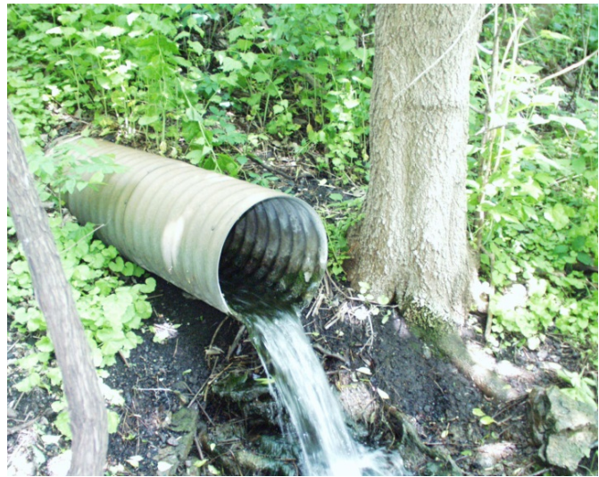
Figure 4 - Flow from Camp Coldwater Reservoir, May 2000
