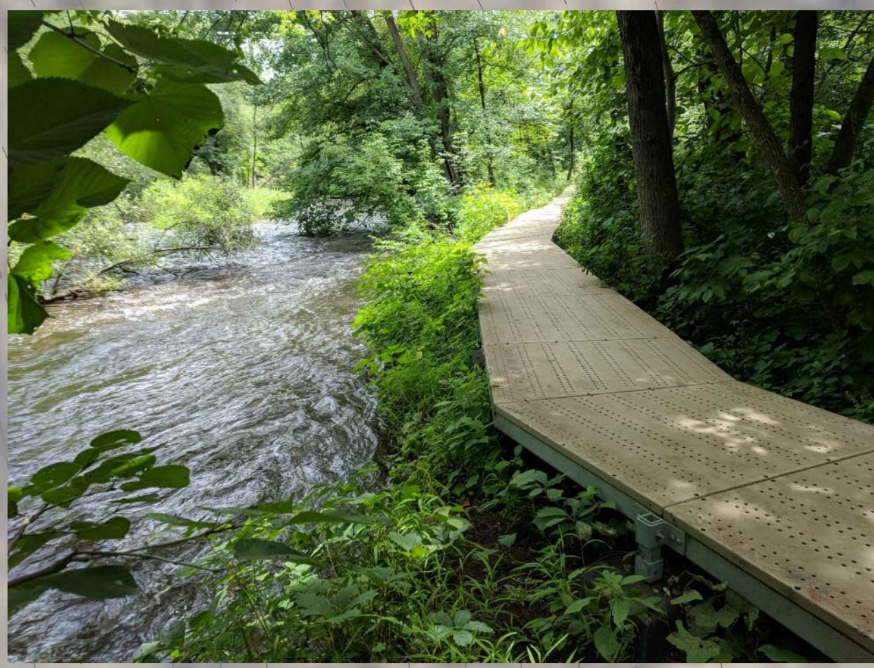
PHOTO - PROJECT 5 LOOKING SOUTHEAST TOWARD PROJECT AREA
