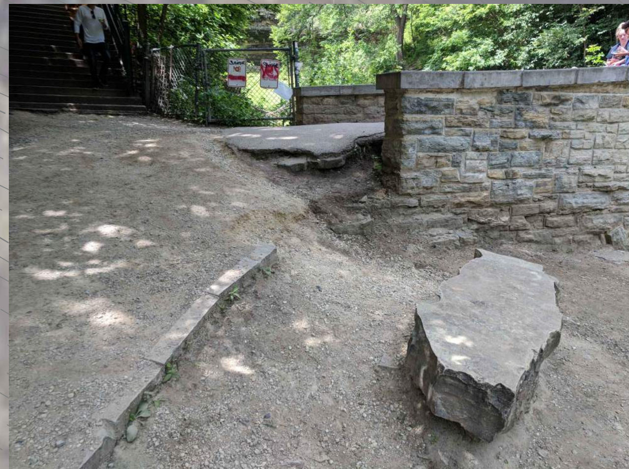
PHOTO - PROJECT 13 LOOKING WEST, TOWARD PROJECT AREA
