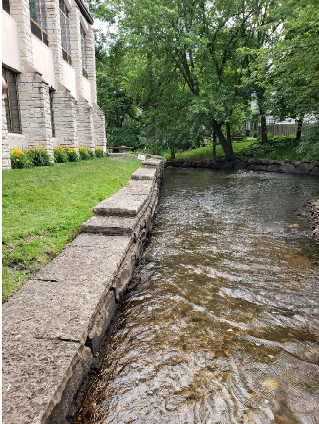
Photo #1 – Interface of retaining wall and creek
