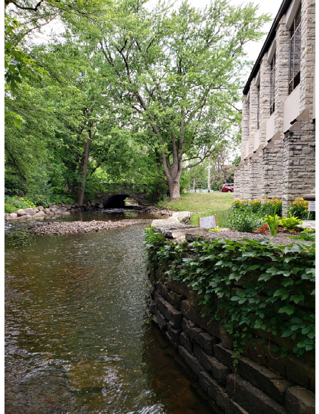
Photo #2 – Interface of retaining wall and creek
