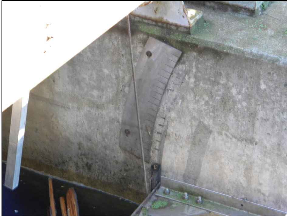
Metal Veneer Bolted to Concrete in Each Bay
