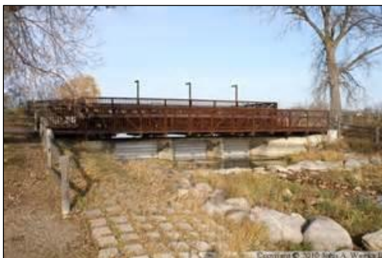
Post-2005 appearance of the dam. Stop logs are installed
