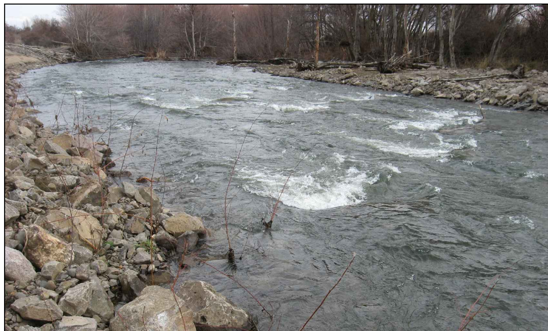
EXAMPLE OF 1.3% ROUGHENED CHANNEL
