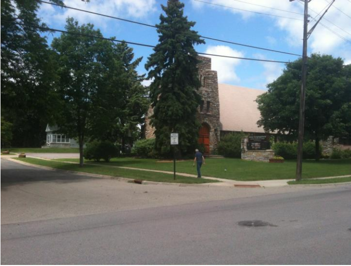
Photo taken from corner of Alabama Avenue (through street to right) and Oxford Street (to left). Entrance to Union parking lot is on left side of picture.
