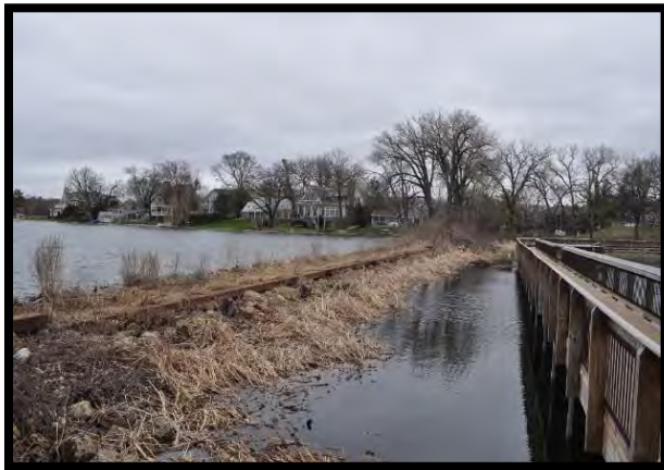
Emergency Spillway May 1, 2014
