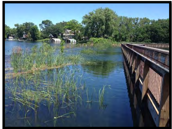
Emergency Spillway June 20, 2014
