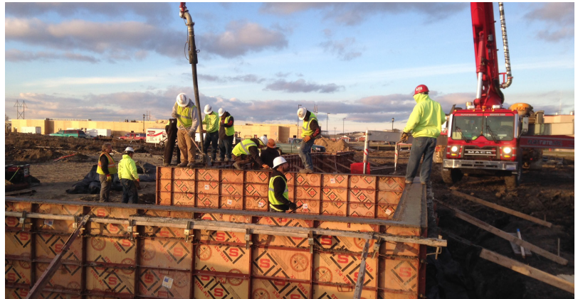
Wenck ensures safety is a priority on all Construction projects.
