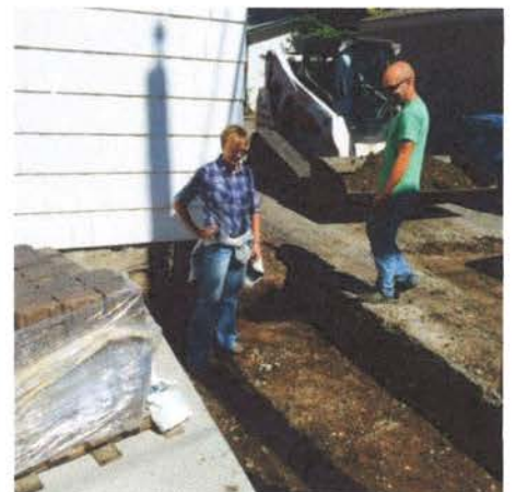
7 excavation for permeable pavers
