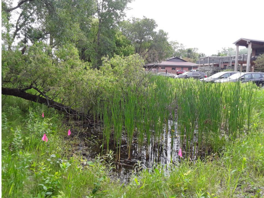
Stormwater pond, facing east.
