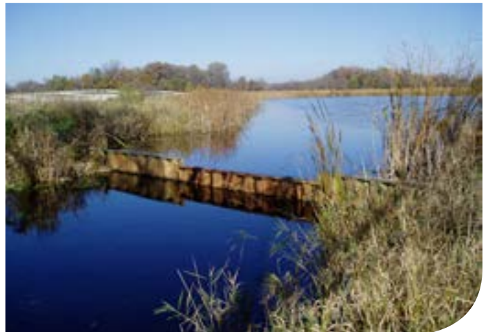
Painter Creek weir
