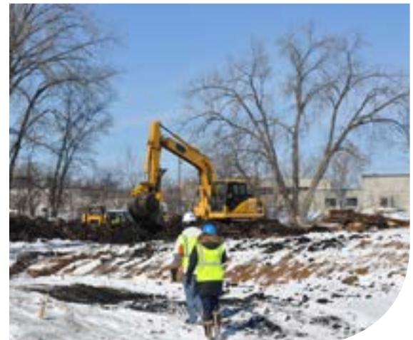
Staff inspecting a construction site
