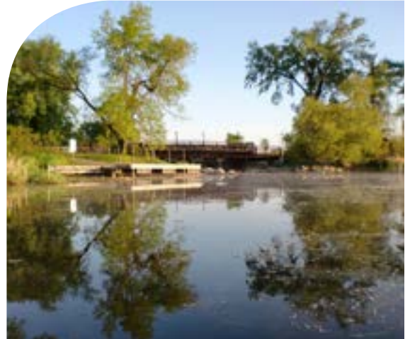
Grays Bay dam, Dale Antonson
