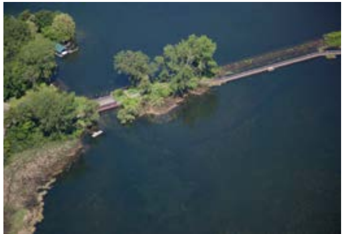
Gray's Bay Dam
