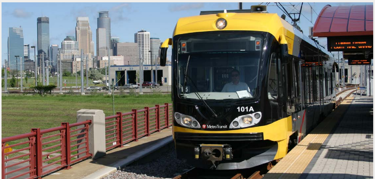
Existing Hiawatha (Blue Line) LRT station with views of downtown
