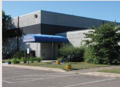
43 Hoops/County-owned development site
