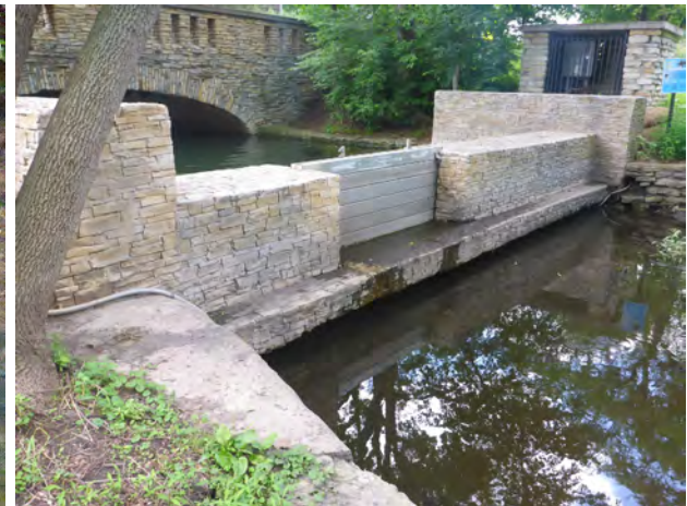
Figure 4. Rebuilt outlet of Lake Nokomis.
