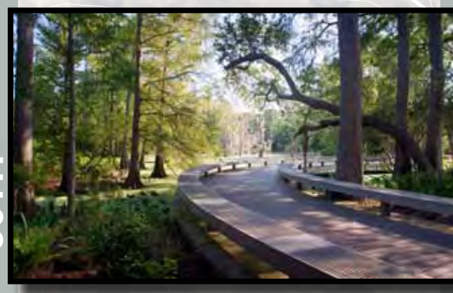
STORMWATER WETLAND WITH BOARDWALK
