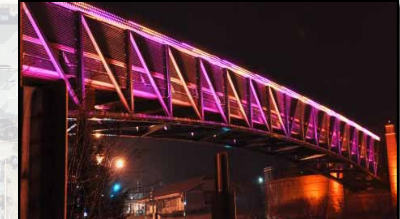
Opportunities for creative art installations at Dupont and Bryant Bridges
