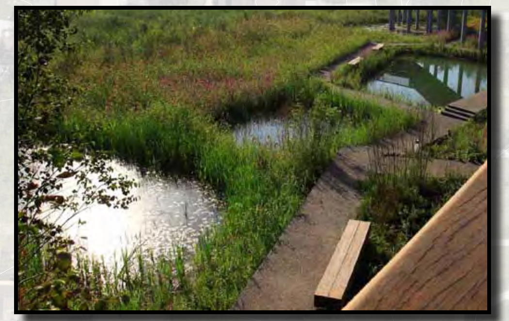
STORMWATER BMP MULTI-CELL BMP (CASCAING POOLS) AND WITH TRAIL OVERLOOKS ALONG THE PERIMETER WITH INTERPRETIVE ELEMENTS INTEGRATED
