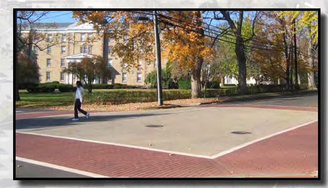
SPEED TABLE: RAISED INTERSECTION WITH HIGH VISIBILITY CROSSWALKS TO SERVE AS TRAFFIC CALMING
