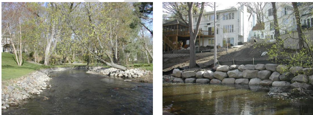
Figure 5: Example of current bank conditions at site
