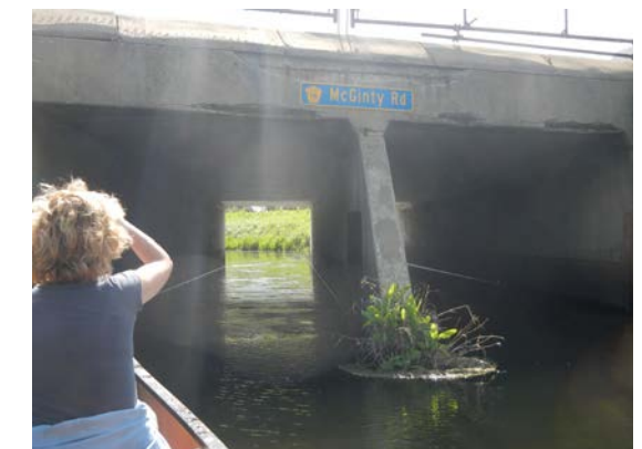
36 Minnehaha Creek Bridge Crossing McGinty Rd & Minnehaha Creek
