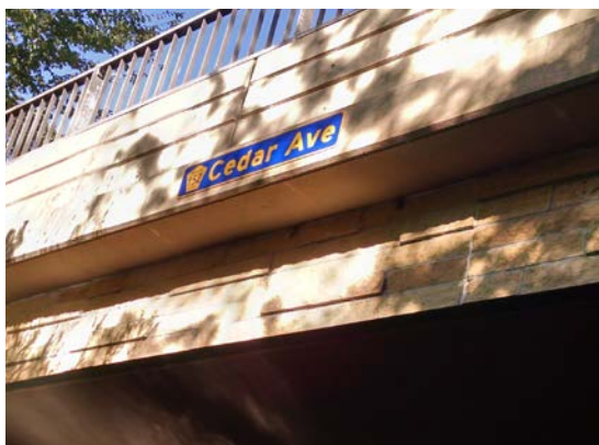
69 Minnehaha Creek Bridge Crossing Cedar Ave
