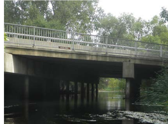
50 Minnehaha Creek Bridge Crossing Louisiana Ave
