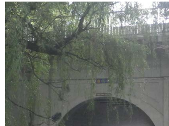
43 Minnehaha Creek Bridge Crossing (2 signs) Minnetonka Blvd
