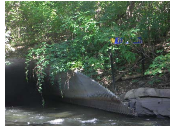
67 Minnehaha Creek Bridge Crossing France Ave
