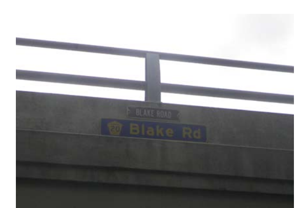
48 Minnehaha Creek Bridge Crossing (2 signs), Blake Road
