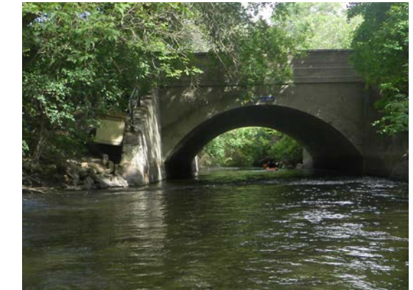
68 Minnehaha Creek Bridge Crossing Xerxes Ave
