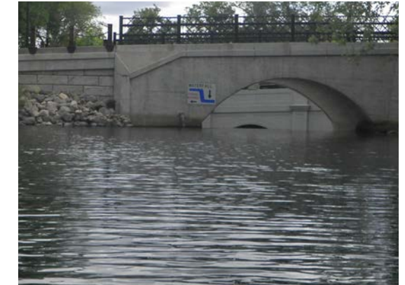
56 Minnehaha Creek Hazard - Waterfall, Browndale Dam
