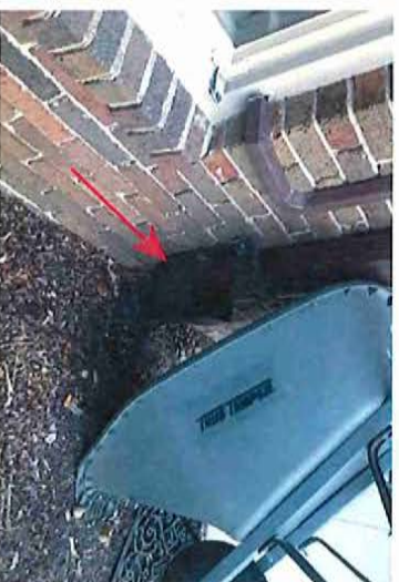
One of the building's downspouts emptying underground.
