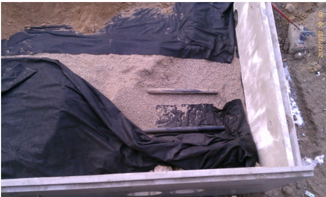
6-inch butt-fusion welded perforated drain tile in filter aggregate prior to slip-joint swivel connection to pending manifold pipe in Mill Street filtration basin.
