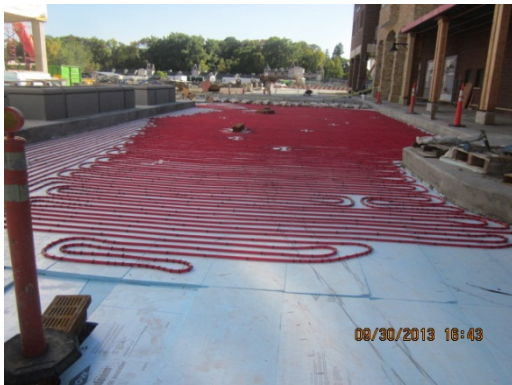
Hydronic snow-melt tubing placed in street during Phase 1 of the project.
