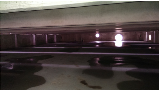
Looking south inside Engel Street detention vault during construction. Two large sun-filled round openings on right are for pending inlet pipes from project roof collection networks. Smaller higher opening on left is opening for eventual overlying street runoff collection pipe to route this dirtier runoff to the Mill Street filtration system.
