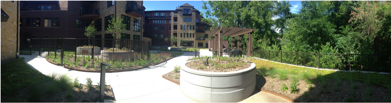
The Terrace green roof of the Folkestone Terrace North (fka, North Block).
