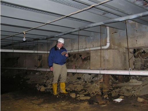
Inspector in “crawl space” below existing mall. Grade level is estimated to have settled about 5-feet since original mall construction in 1964. AET, Inc.
