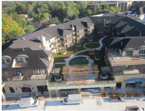
Recently completed green roof of the Folkestone Terrace West (fka, Superior Block). Photo courtesy of Adolfson & Peterson Construction.
