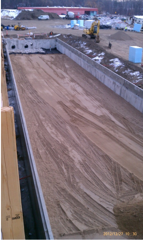
Recently placed clean sand in the Mill Street filtration basin prior to covering with sacrificial filter fabric and capping the basin with precast double tee structural members (left – looking easterly, right – looking westerly).
