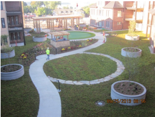
Recently completed green roof with putting green on the Folkestone Terrace West (fka, Superior Block). Photo courtesy of Adolfson & Peterson Construction.
