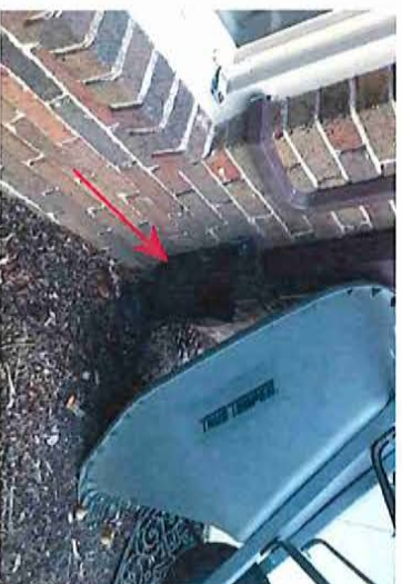
One of the building's downspouts emptying underground.
