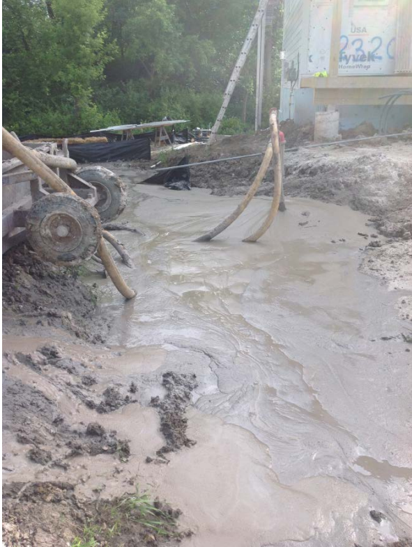
Site condition documented on 6/8/18
