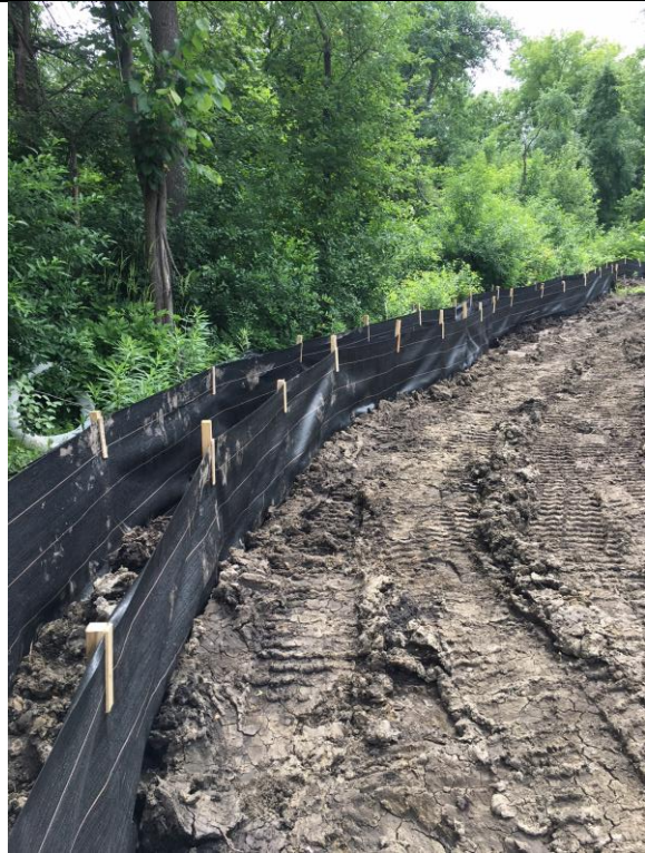
6/25/18: Re-grading and redundant silt fence as a response to spill
