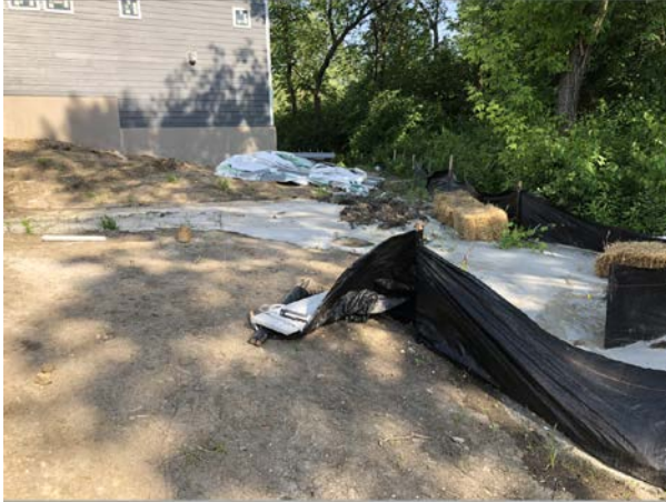
Site condition documented 6/15/18
