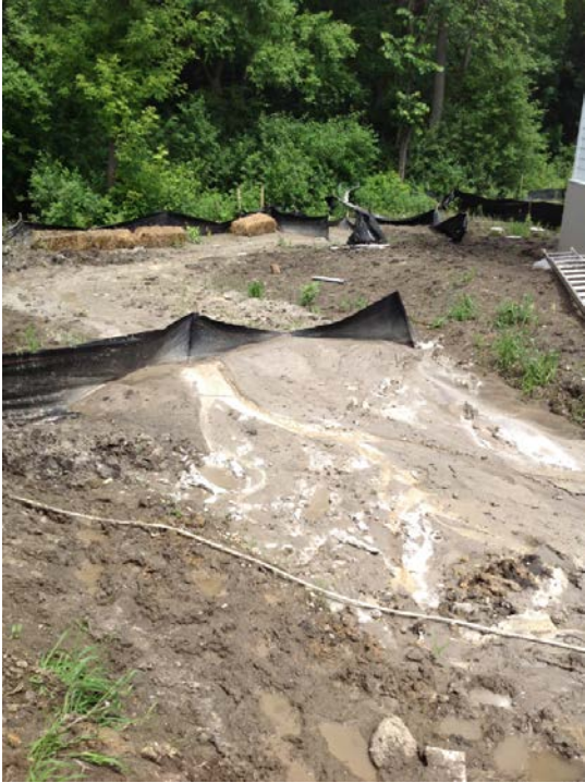
Site condition documented 6/20/18
