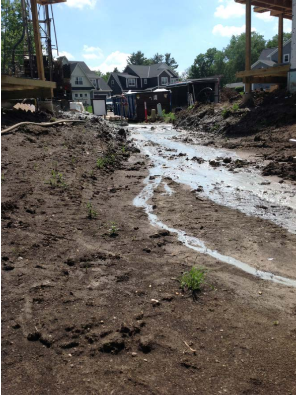
Illicit Discharge flowing through site 5/31/18
