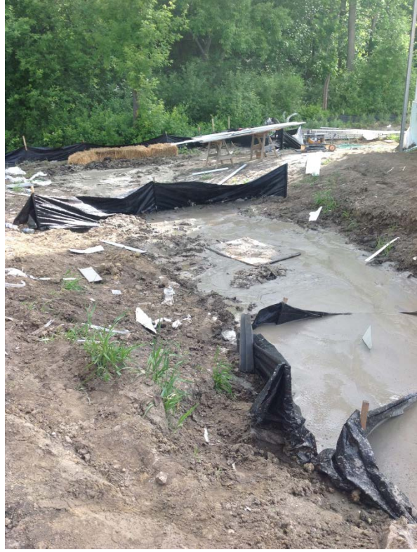
Site condition documented on 6/8/18
