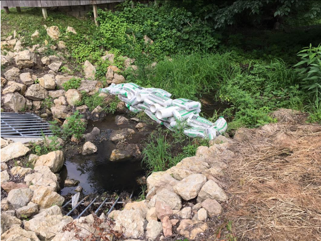
6/25/18: Underflow dam at Watertown Road preventing downstream migration of bentonite material.
