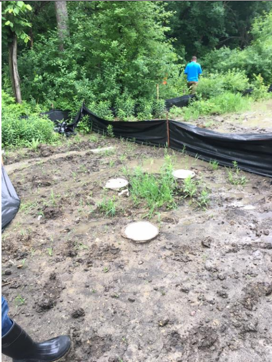
6/19/18: Silt fence in place at development
