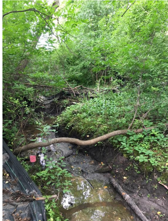
6/25/18: Clean-up efforts; silt fence in need of maintenance
