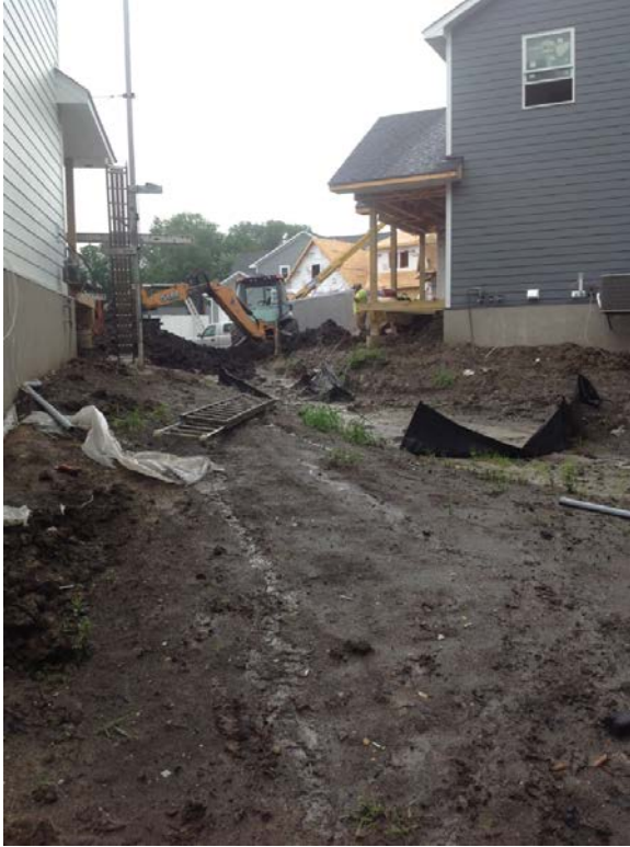
Site condition documented 6/18/18
