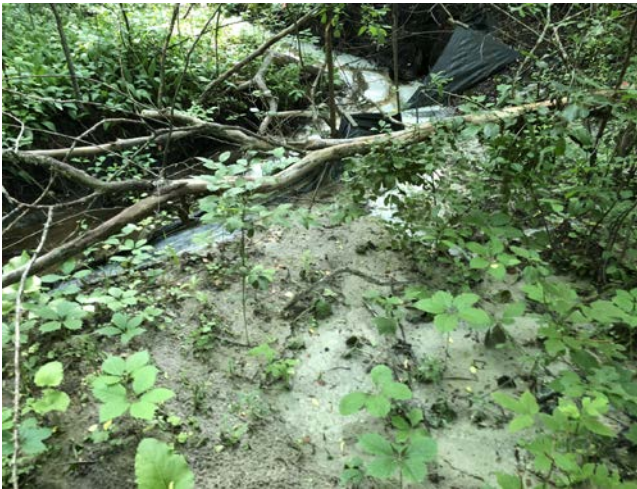
Failing Erosion Control and illicit discharge within stream documented 6/15/2018
