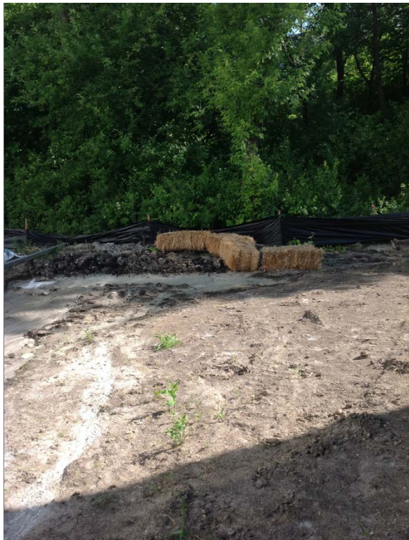
Perimeter control documented on 6/5/18
