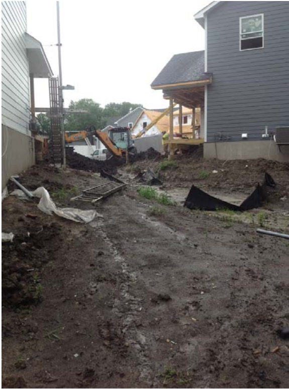
Site condition documented 6/18/18
