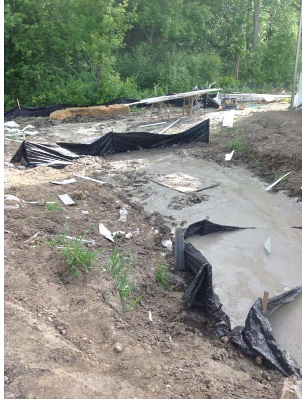
Site condition documented on 6/8/18
