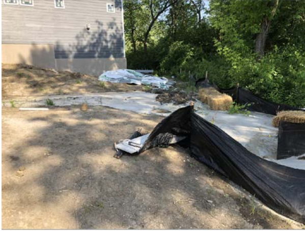
Site condition documented 6/15/18
