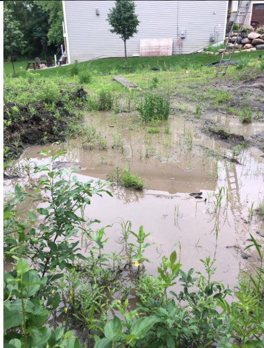
6/19/18: Bentonite pooled at well site/development
