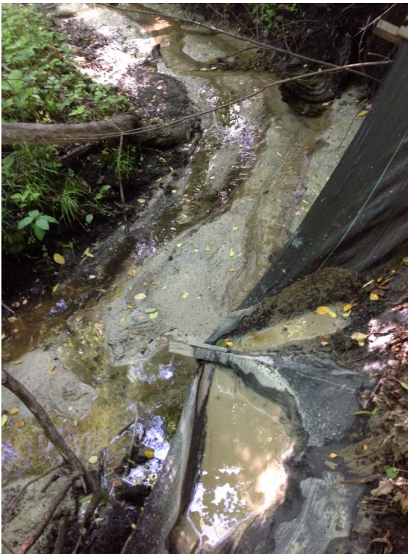
Illicit Discharge in stream and failing erosion control documented on 6/5/18
