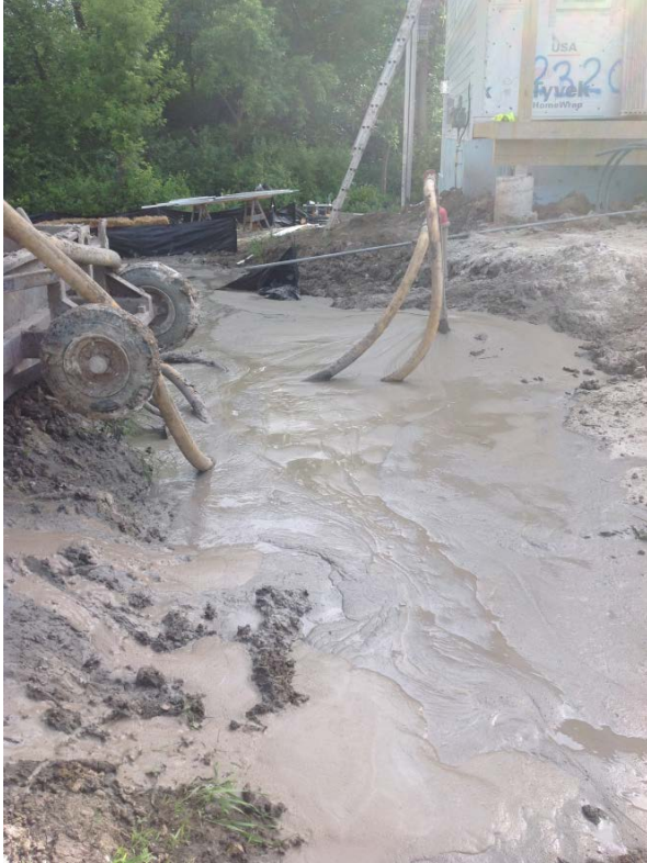
Site condition documented on 6/8/18
