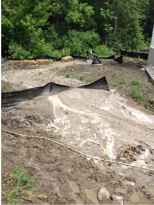
Site condition documented 6/20/18
